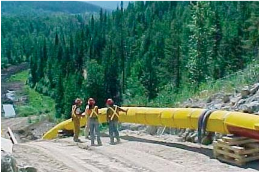
Pipe: 24" Custom Cut Pads. Size 80" x 72"
